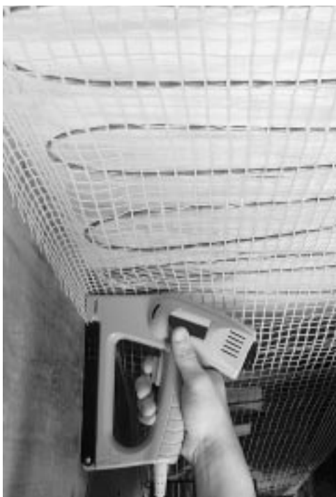
Stapling SunTouch UnderFloor mat to floor joists.
