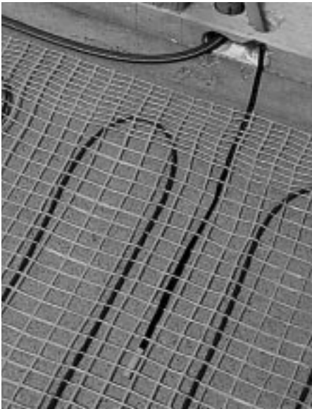
Bottom plate/sensor detail. Simply “weave” the sensor into the mat, or you may prefer to use a clip.
